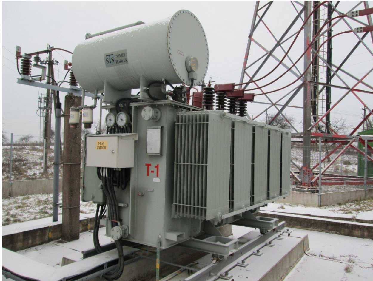
10 MVA Power Transformer in Lithuania
